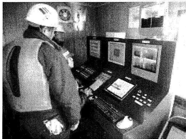
Figure 9 Remote monitoring and controlling installation work
