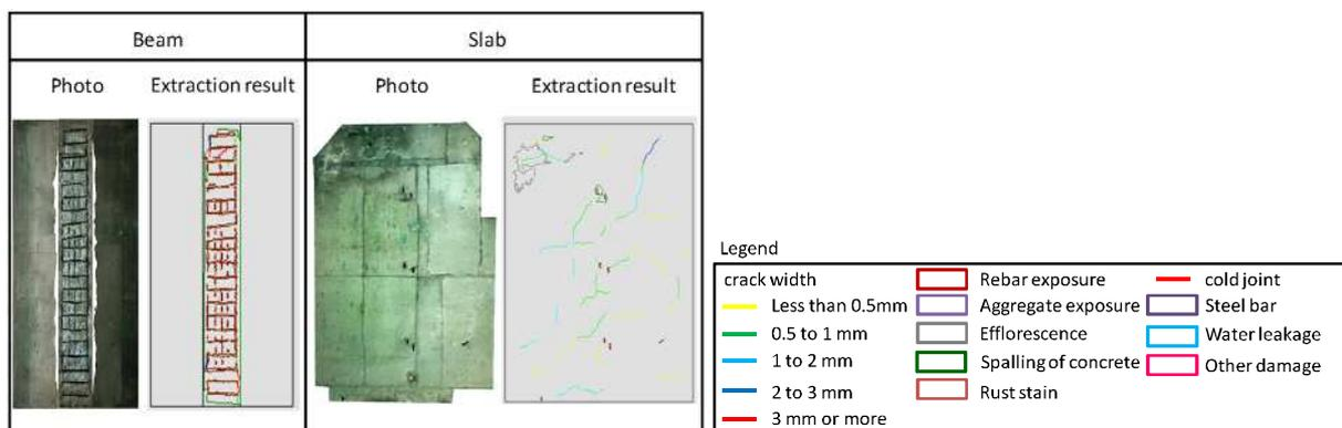
Figure 4.8: Enlarged orthochromatic images and drawings resulting from extracting degradation
