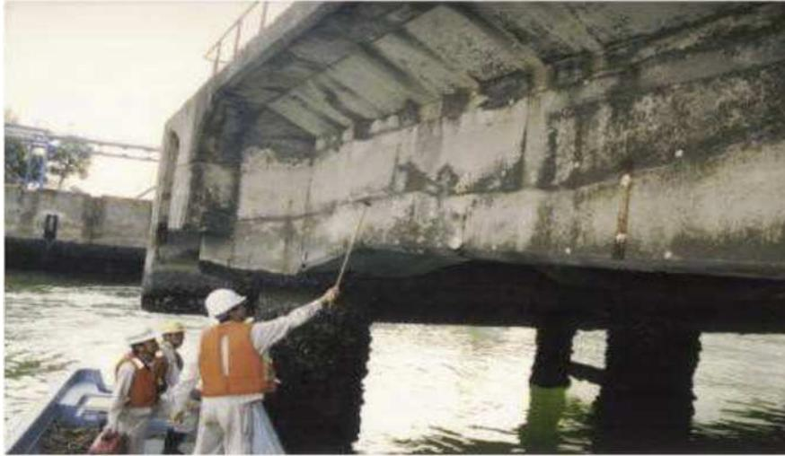
Figure 1.1: Investigation of the undersurface of the superstructure of a piled pier (conventional method)
