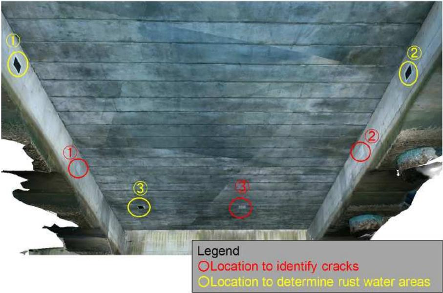
Figure 3.8: 3-D model of the examined piled pier
